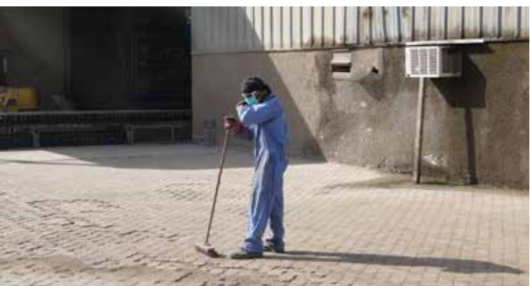
Sweeping and collecting dust from paved areas is a common control measure to reduce the amount of dust that can be re-suspended into the air from trucks and wind.
